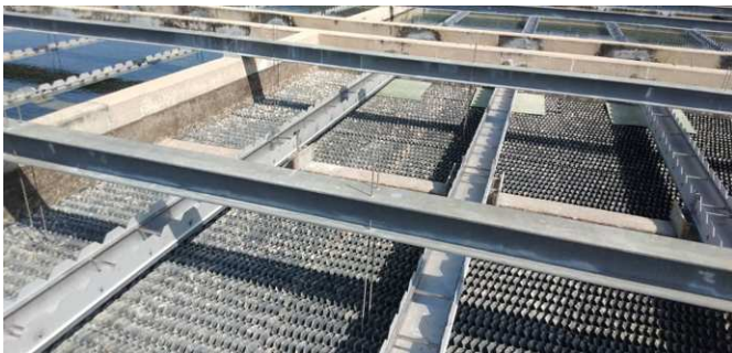
Replacement of stainless steel trough at Plant B Johor River Waterworks.
