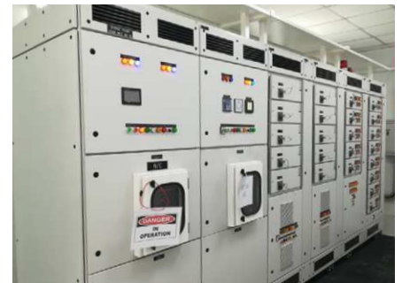
Replacement of 6.6kV Switchgears, 415V switchboards, transformers, cables and ancillaries at Johor Plants.
