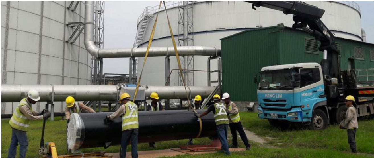
Overhaul of Pumps in Catchment & Waterways.
